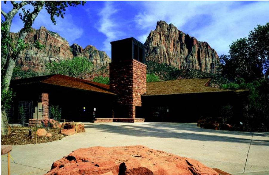
Photograph courtesy of DOE/NREL
